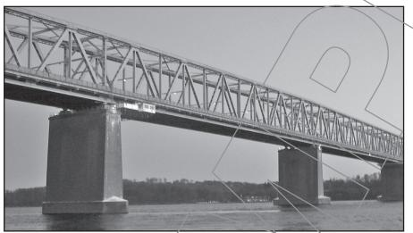
A **truss** is a structural frame made of straight beams in the shape of a triangle.
